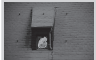
Example of the fire in the roof framework. The roof is still intact outside. Thereby there was to fight against no possibility the fire.
