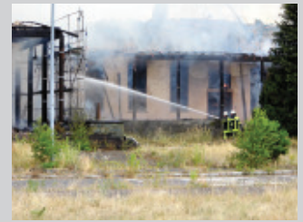
Firefighting on the front of the building
