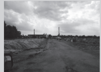
Pictures of the construction site from 2014
