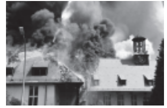
The fire broke out in the central roof area of the building from
